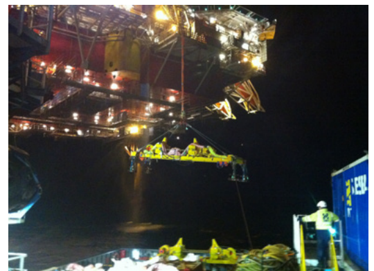
Deployment of Sling Tensioners from Diving Support
