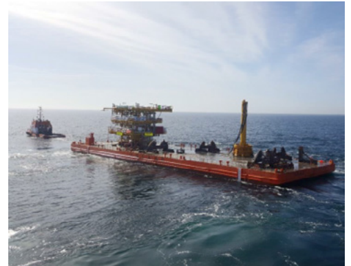
Transport of tower and monopile prior to installation
