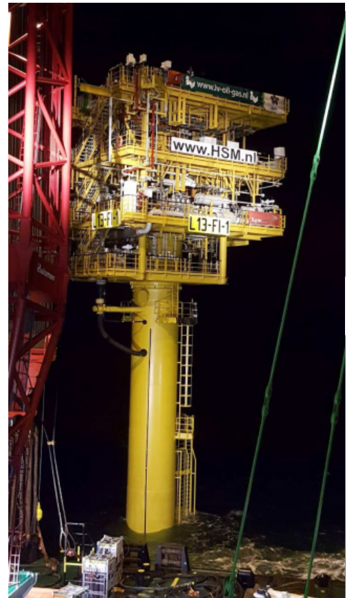
Installation during night
