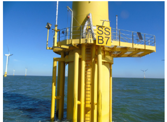
Scroby Sands Offshore Windfarm
