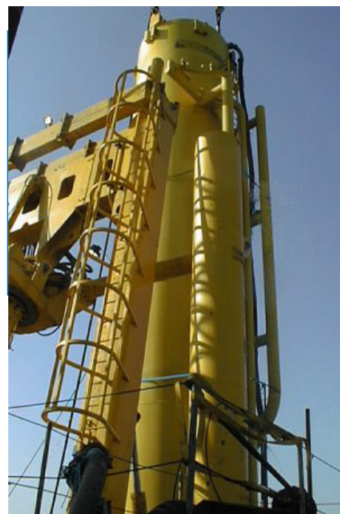
Scroby Sands Offshore Windfarm - Installation
