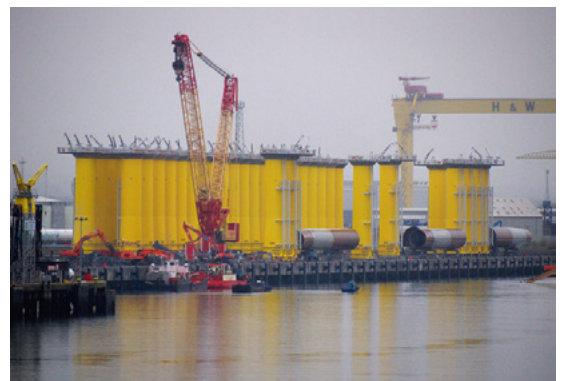
Monopiles ready for commissioning
