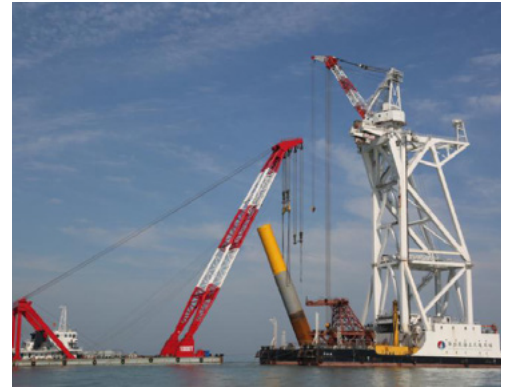
Installation of DAFENG H3 offshore Windfarm, China
