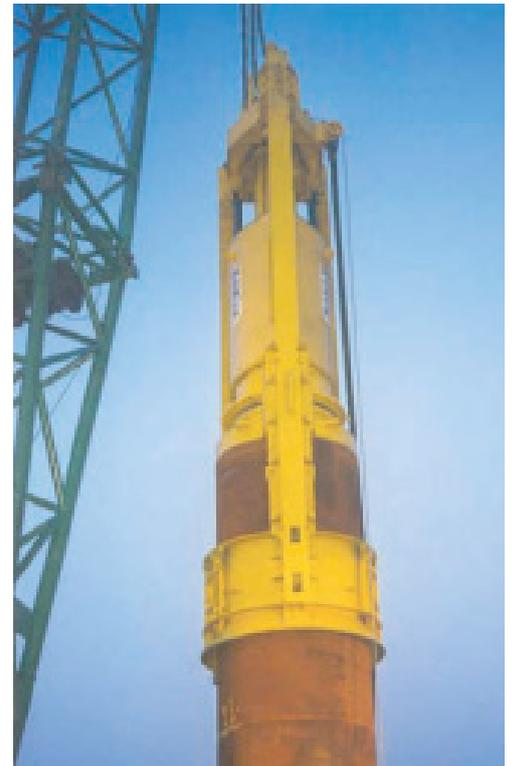
Driving of Ø1620 mm monopile at Horns Rev
