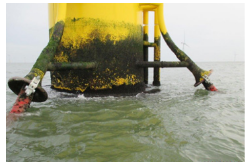
Reinstatement clamp fitted to bellmouth on the site
