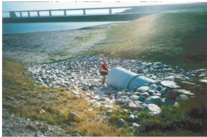
Scour Protection of Outlet from Storm Surge Relief Culvert. Great Belt Link, 1995.
