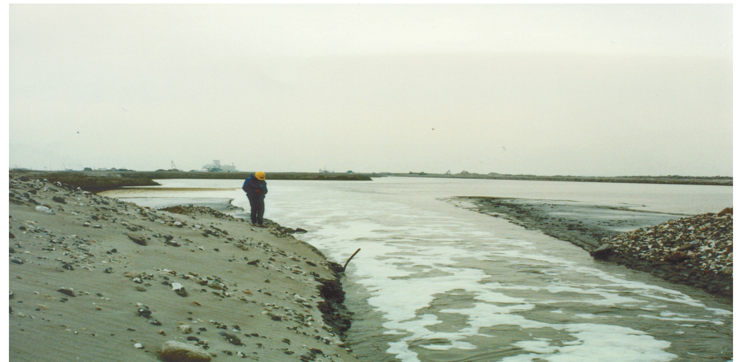
Picture above shows open channel carrying sediments in very high concentrations. The channel was designed to be completely self-cleaning under all flow situations, including temporary stops. Great Belt Link.
