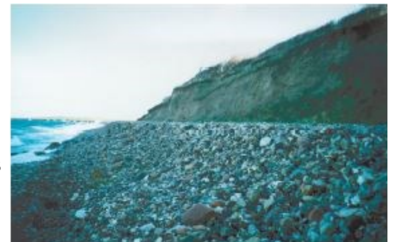
Scour protection of cliff by pebble revetments. A "natural appearance" is obtained together with a sufficiently strong beach profile. Sprogø 1996-97.
