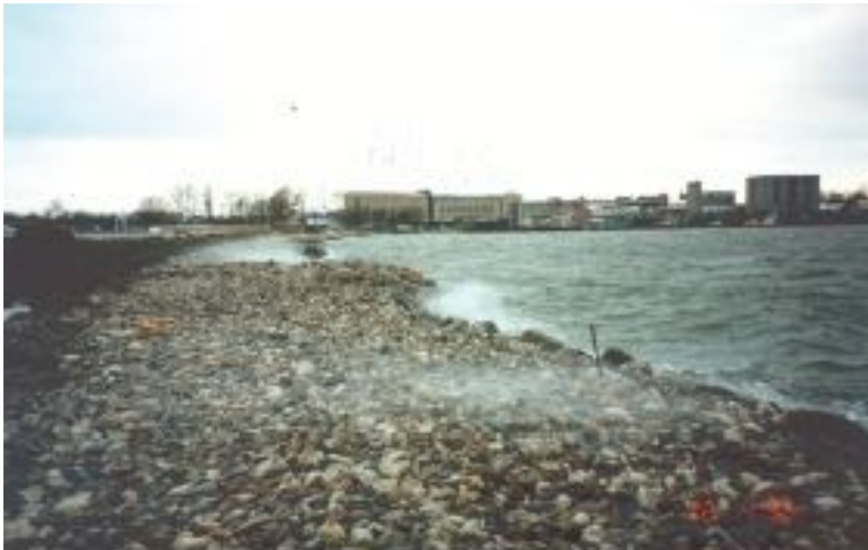
Scour protection in coarse pebbles. Øresund Fixed Link, 1995.
