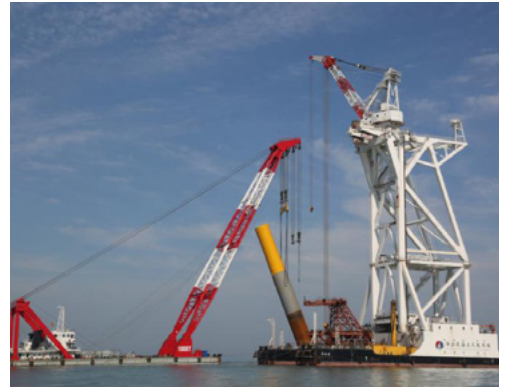
Installation of DAFENG H3 offshore Windfarm, China
