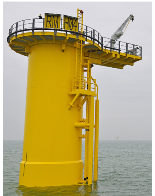
Rampion Offshore Windfarm
