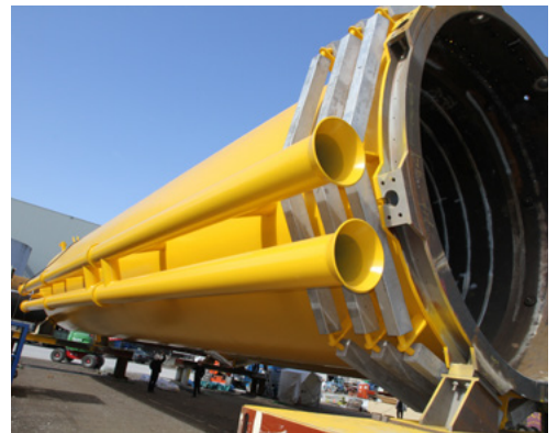
Monopile for Northwind, ready for installation
