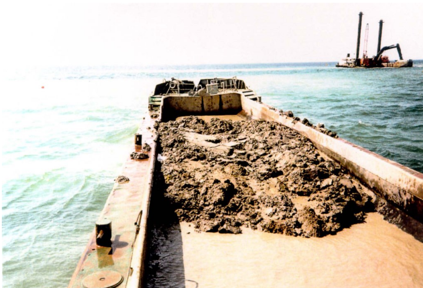
Trial dredging by the hydraulic dredger "Rocky"
