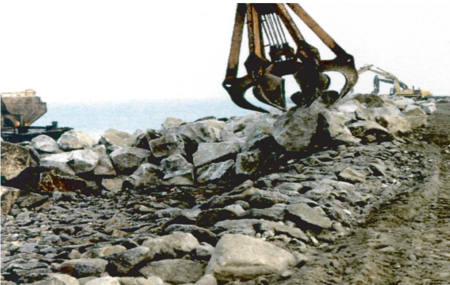
SPROGØ: Placing of armor stones
